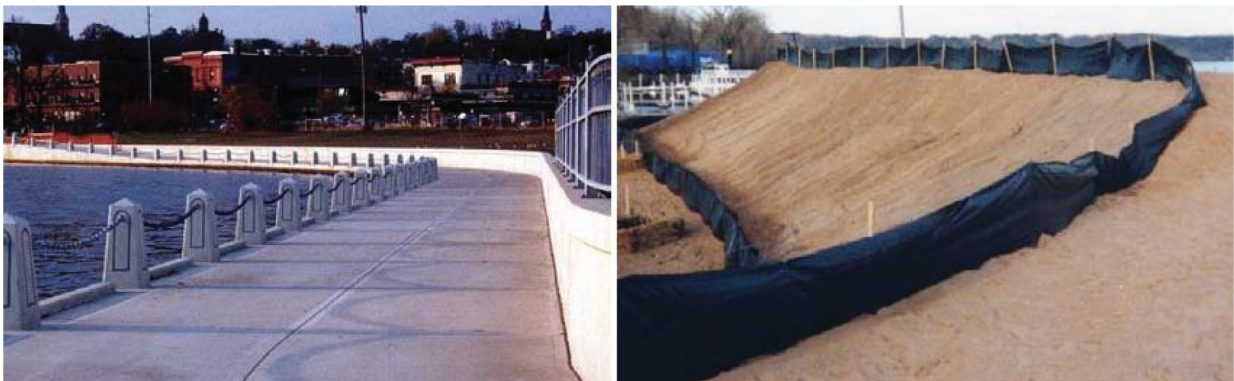
Stillwater Flood and Retaining Wall Project, Minnesota
